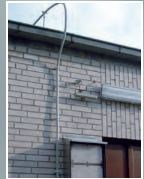
System DEHNconductor - vodič HVI®
