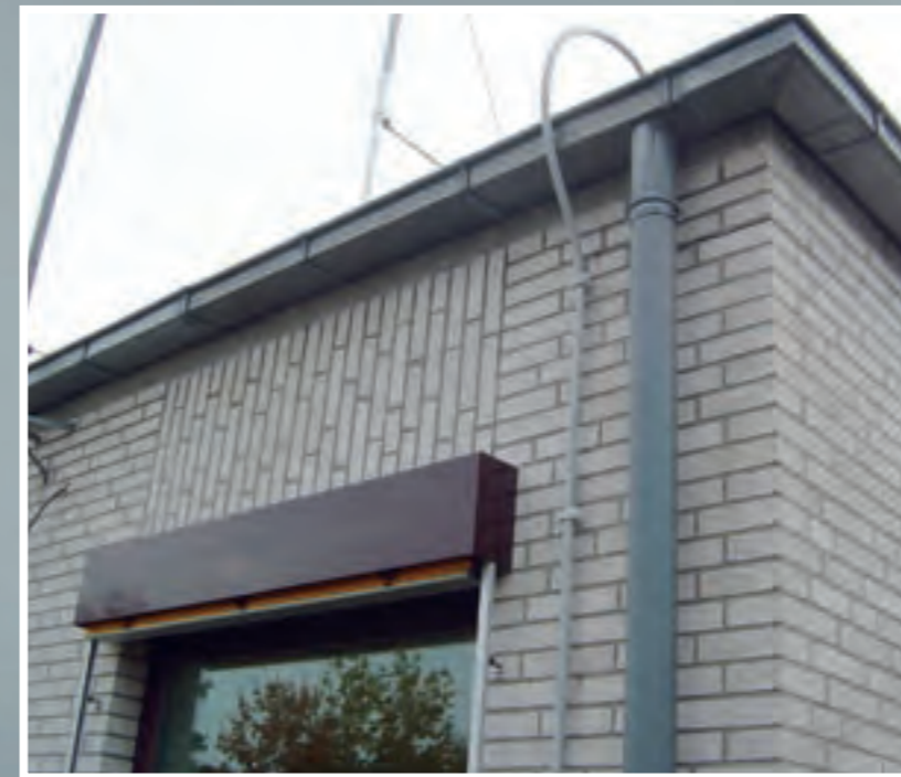
System DEHNconductor - vodič HVI®
